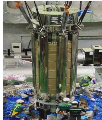
CS under Installation
